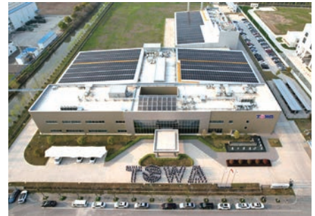
Solar panels installed at the Nantong Plant
