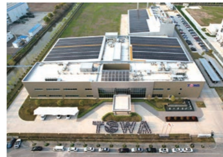
Solar panels installed at the Nantong Plant
